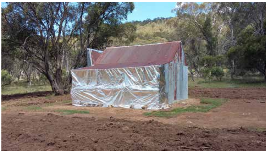
Bill Jones Hut was wrapped in thermafoil and had an earth break constructed around it for fire protection.
